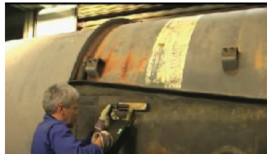
Removal of hard and soft vulcanized rubber (from 12000 to 15000 microns)
