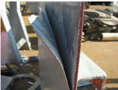
Removal of fire retardant coatings such as Chartek (from 8000 to 13000 microns)
