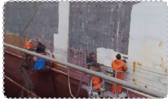
Ship Hull - Gothenberg, Sweden, February 2008. Removing epoxy coating.
