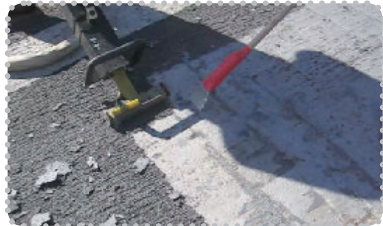
Aircraft Carrier - US, May 2007. Removing anti-skid deck coating. Epoxy with carborundum grit. 2000-3000 microns
