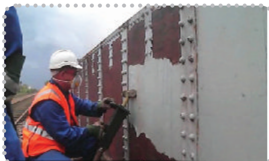
Railroad Bridge - UK, June 2007. Removing epoxy paint. 400-600 microns with iron oxide primer
