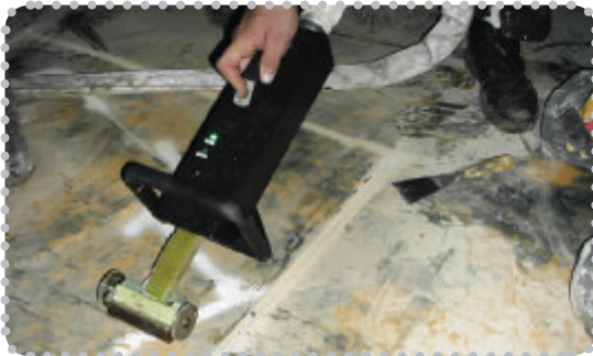
Chemical Tank - France, June 2007. Removing tank bottom lining. Fiberglass reinforced epoxy. 1500-2000 microns
