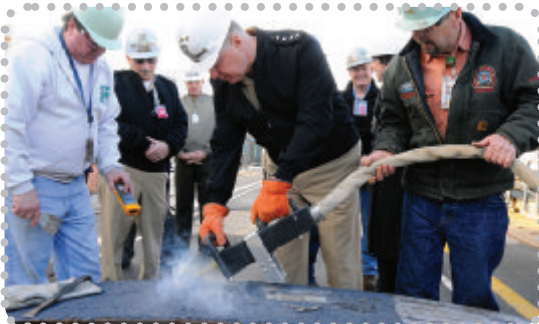
Naval Shipyard - US, January 2008. Removing various coatings including rubber and anti-skid.
